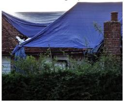
As you see from the photograph, the roof has recently been covered by a tarpaulin after a year of exposure to the weather. However by the 30<sup>th</sup> July (within a fortnight) the west side was once again adrift and the roof exposed to the weather. We are pressing for ABC action again.
